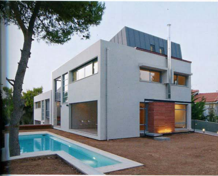
On the south side, two loggias link the living areas and the garden area, which is characterised by a reduced design.
